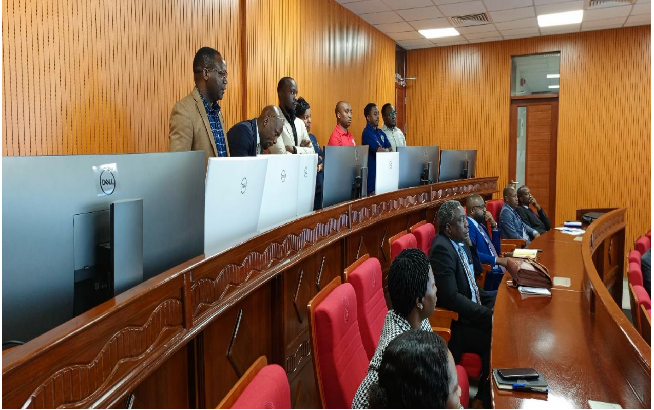
Laptop Computers at the Back of the Situation Room that project the Information that is seen at the Display Screens
